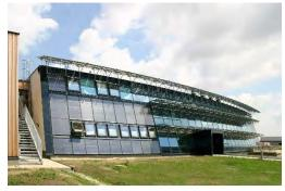
Fig. 6 Façade-integrated Photovoltaic panels, Photo Credits: Architekturbüro Reinberg ZTGmbH
