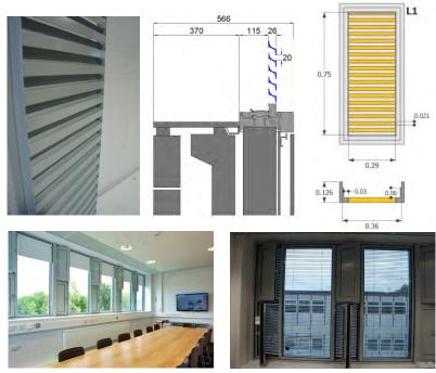
Fig. 10 SLOTTED LOUVRE VENTILATION COMPONENT
