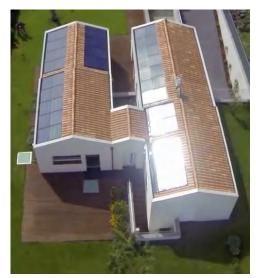
Fig. 6 PV PANELS AND SOLAR THERMAL PANELS
