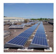
Fig. 7 INSTALLED PV ARRAY ON ROOF OF EXISTING BUILDING
