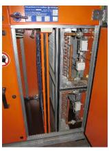
Fig. 7 HEATING COILS IN THE AIR HANDLING UNIT
