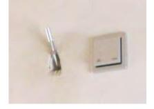
Fig. 17 EXAMPLE OF INDOOR SENSOR INSTALLED TO MEASURE TEMPERATURE, RH, CO2 CONCENTRATION
