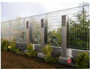
Fig. 10 INLET DUCTS OF THE EAHE
