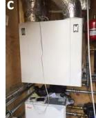
Fig.8a)East side , b)Accumulation tank, c)AHU and heat pump
