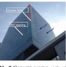
Fig.9 CORNER VOIDS AND AIR INTAKE SLITS IN THE WALL
