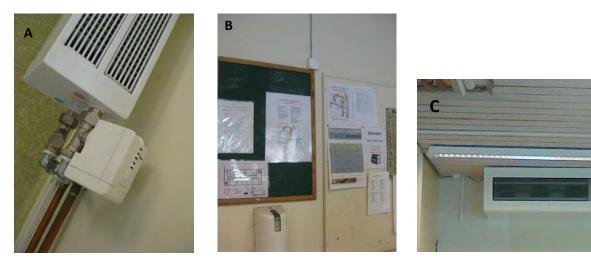
Fig.6 A) DETAIL OF THE CONTROLLER FOR THE RADIATOR, B) DETAIL OF THE PLACING OF THE TEMPERATURE AND CO2 SENSOR C) EXTRACT OPENING FROM THE CLASSROOM
