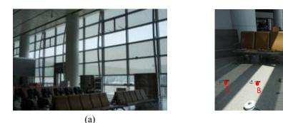
Fig. 4-3 Building envelope of the departure hall: (a) Glass curtain wall; and (b) Solar radiation through the glass on the floor.
