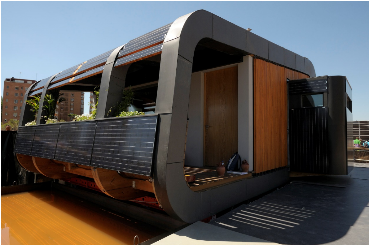
Figure 4-22: The house entitled Urcomante by the University in Valladolid with façade-integrated PV and water basin in the foreground. Source: Solar Decathlon Europe (SDE flickr, 2010)
