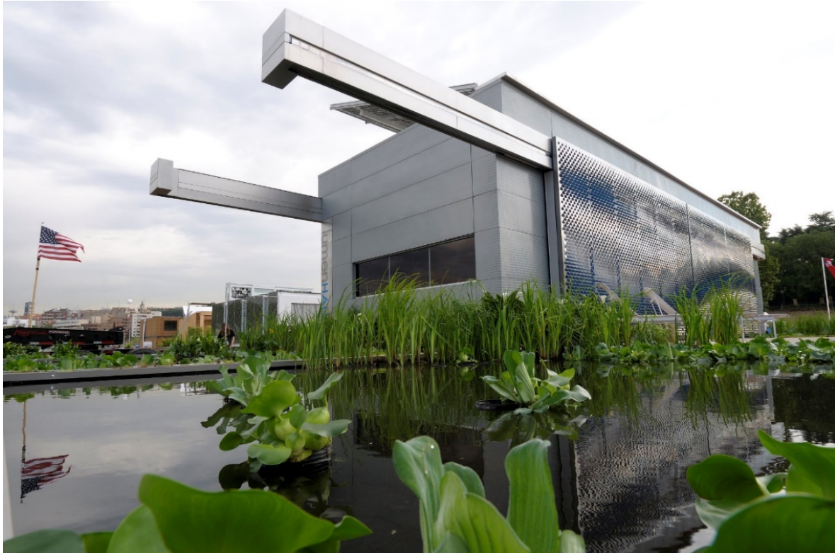
Figure 4-26: Exterior view of Virginia Tech's Lumen House at SDE2010 in Madrid. The house was perfectly designed for transport conditions and can be transported in one piece with all façade and roof cladding. Source: Solar Decathlon Europe (SDE flickr, 2010)
