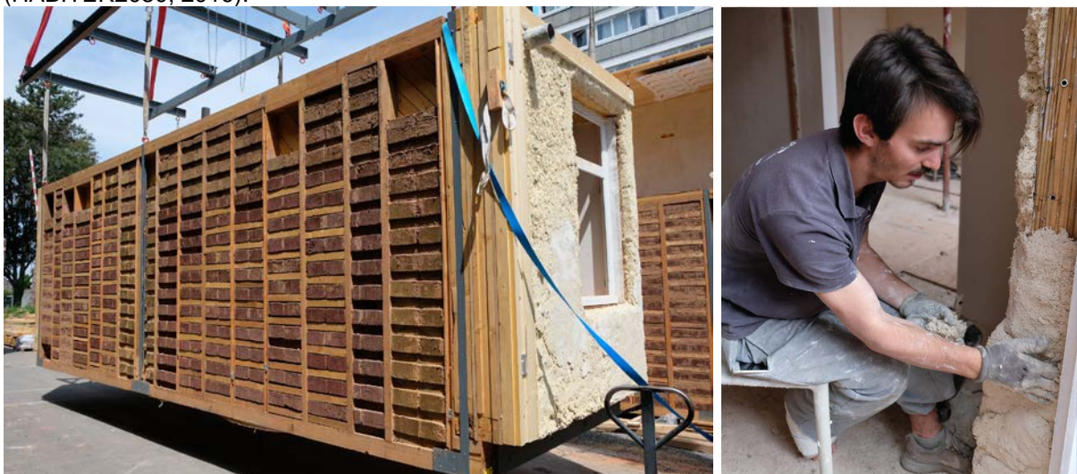
Figure 5-12: Built-in clay bricks and lime-hemp-based underplastering, Source: (HABITER2030, 2019)
