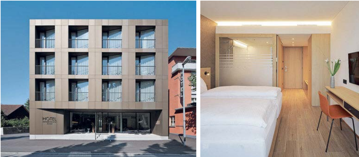
Figure 4-3: The rooms of the Hotel Katharinenhof in Dornbirn were developed as room cells and delivered to the construction site fully equipped. Source: Johannes Kaufmann Architektur, © Radon Photography (Kaufmann et al., 2017, S. 72–73)
