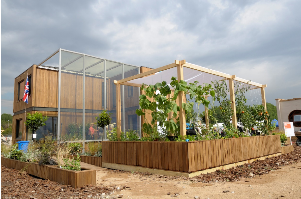
Figure 4-16: Exterior view of the Nottingham H.O.U.S.E at SDE 2010. The team chose to leave the joints between the elements visible and cover them with reversibly fixed moulded metal parts. Source: Solar Decathlon Europe (SDE flickr, 2010)
