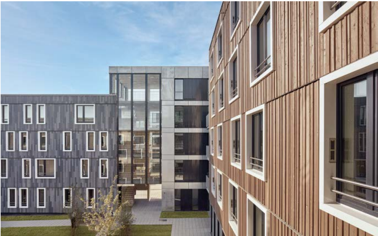
Figure 4-2: Student residence in Bochum, which was developed as a model project of the Zukunft Bau initiative. The building is constructed in elemental reinforced concrete skeleton construction with prefabricated timber panel elements. Source: ACMS Architekten GmbH, Wuppertal, © Sigurd Steinprinz, Düsseldorf (Jakob, 2019, S. 50)
