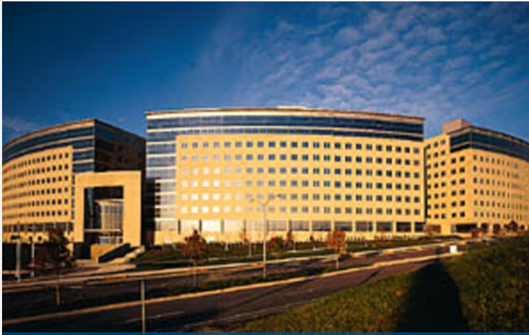
New Carrollton Federal Building
