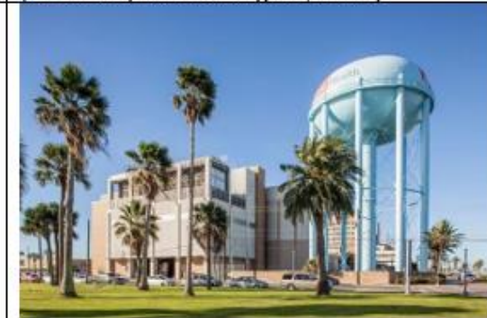
Figure 8.5f Elevated Boilers and Chillers (The University of Texas Medical Branch at Galveston)
