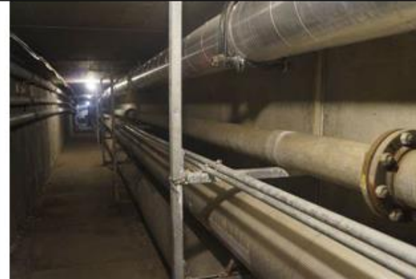
Figure 8.5c. RICE University underground tunnel
