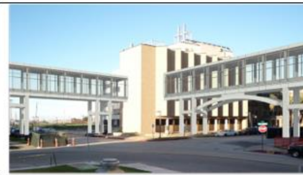
Figure 8.5a Underground steam lines have been replaced by steam lines installed under skyways to research buildings (The University of Texas Medical Branch at Galveston)
