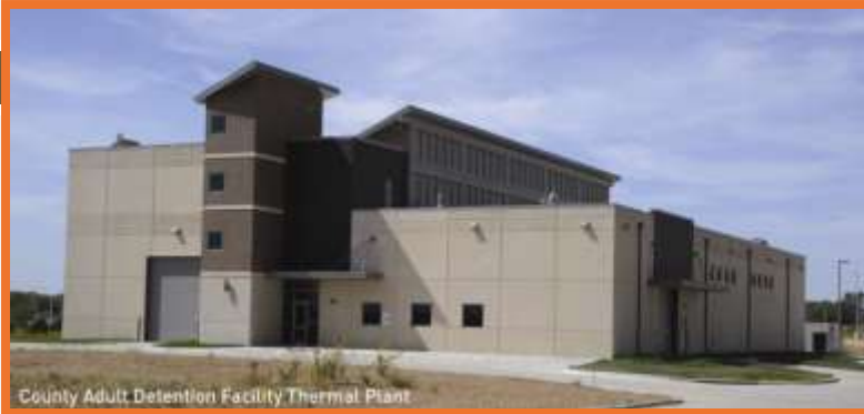
County Adult Detention Facility Thermal Plant
