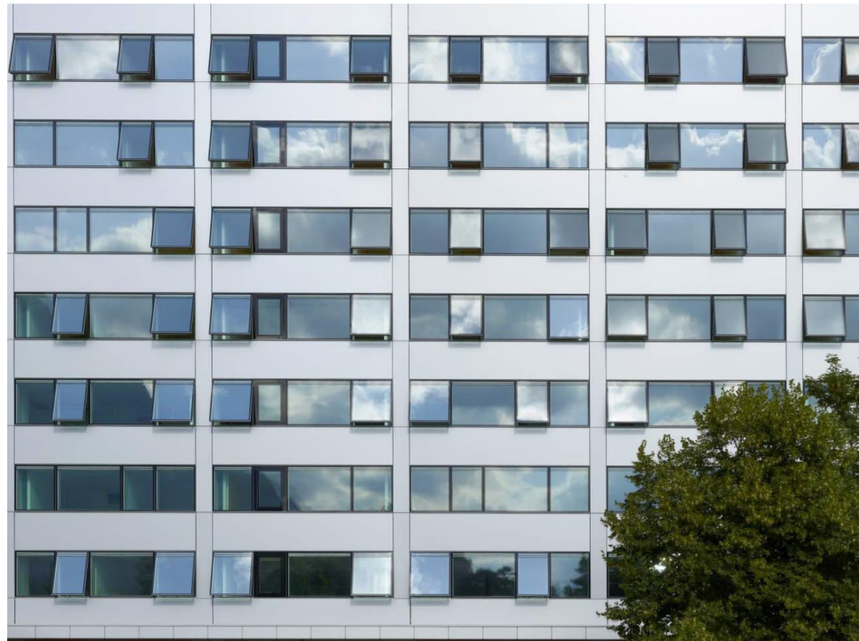
New façade of the building in focus of the renovation. Source: ATP architekten
