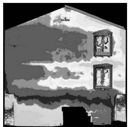
Figure 5: Laser scanning of a demonstration building (left). The measurements show a deformation of a façade of \pm 4 cm (right) that can hardly be detected by traditional measurement techniques.
