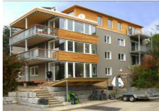
Figure 12. Swiss apartment building in Zurich, before and after renovation with prefabricated roof and façade elements. The renovation includes a new attic floor, living room extensions with old balconies, new enlarged balconies.
