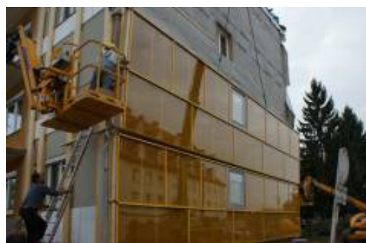
Figure 9. Mounting of pre-fabricated roof and façade elements .
