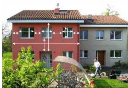
Figure 8. Photogrammetry allows for normalisation of digital photos, which can then be used for measurement extraction.
