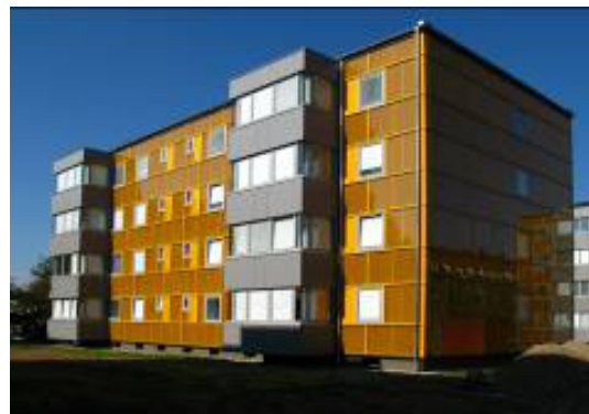
Figure 13. Austrian apartment building in Graz, before and after renovation with prefabricated façade elements. The renovation includes solar façade elements, living room extensions with old balconies, new elevators.
