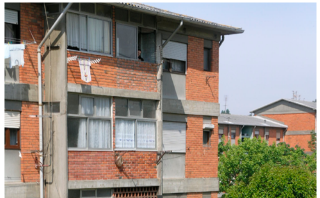
Social housing in Porto, Portugal Source: Vasco Freitas
