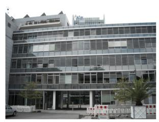
Figure 2-38: Two-part sun protection enables glare-free use of daylight
