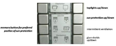
Figure 2-41: Control device and its functions
