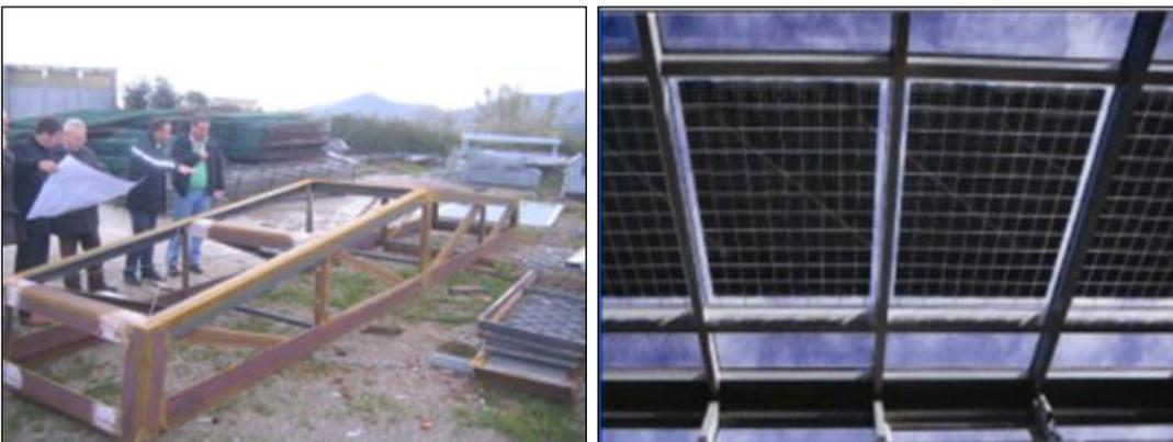
**Figure 7.116. Structure for the glazed roof and semi-transparent PV cells.**
