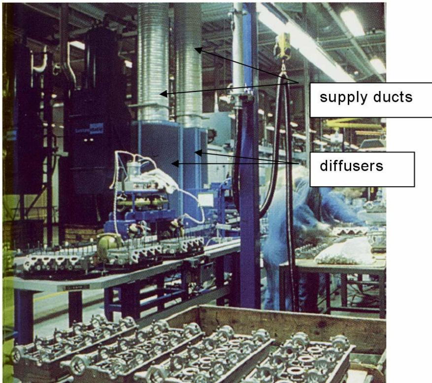
Figure 6.20. Industrial displacement ventilation system.
