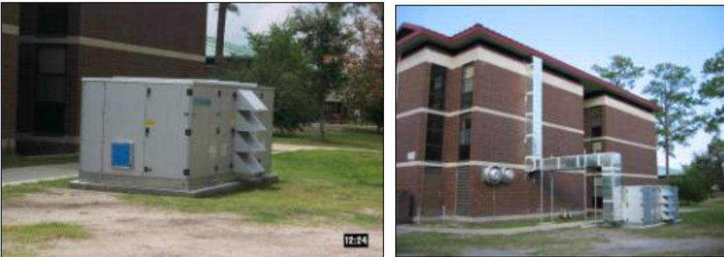
Figure 7.73. Blue rectangular opening is the location of (future) supply duct connection. Completed system is shown at the right.
