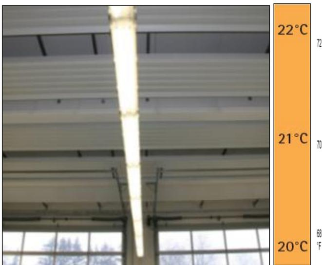
Figure 7.127. The new radiant power heating keeps the temperature more constant between the floor and ceiling.
