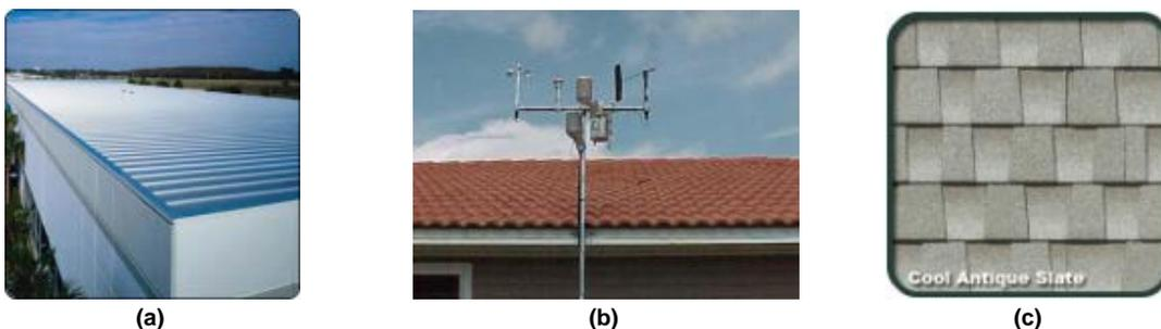
**Figure 6.4. White metal roof (a), roof tile coatings (b), and architectural shingles (c) (<http://www.elkcorp.com>).**
