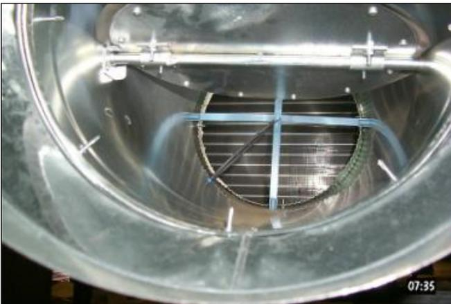
**Figure 7.56. Airflow measurement sensor and motorized damper downstream of reheat coil.**
