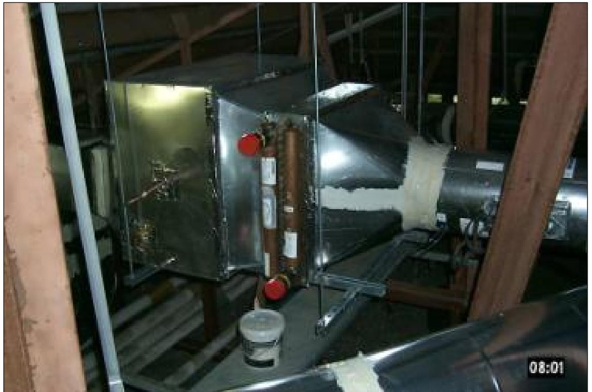
Figure 7.54. DX cooling coil located to the left. Hot water reheat coil shown in the center. The motorized damper actuator is barely visible behind the steel framing member to the right.
