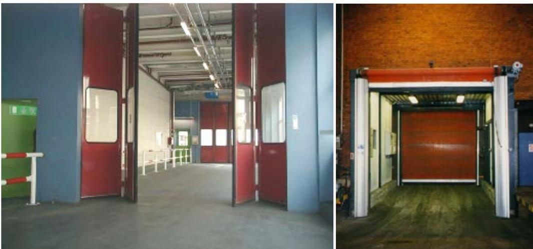
**Figure 6.91.** Examples of large industrial facility doors protected by a vestibule.
