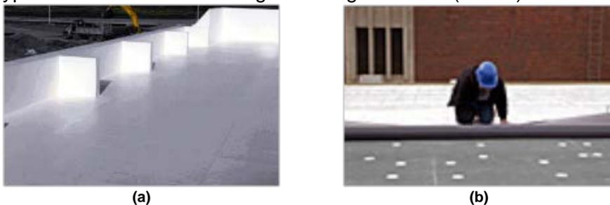
**Figure 6.3. Reflective roof coating (a), and reflective roof membrane (b).**
