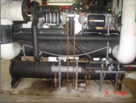
**Figure 7.139. Oil-free magnetic bearing chiller compressor.**
