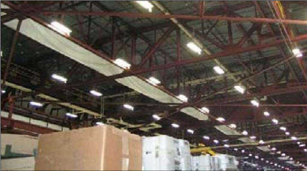
**Figure 7.132. Ventilation air distribution ducting.**
