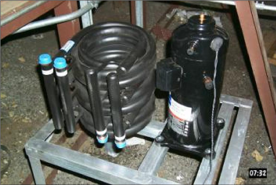
**Figure 7.55. DX compressor and water-cooled condenser.**
