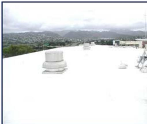
**Figure 6.2. Duro-Last Cool Zone® roofing system with a single-ply, 40 mil membrane roofing material and a polyvinyl chloride polymer blend demonstrated through the Navy Technology Validation (Techval) Program.**
