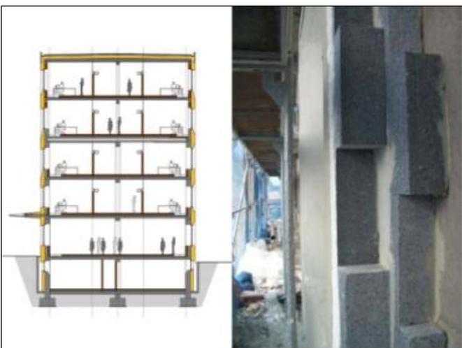
**Figure 7.10.** Section and picture illustrating the insulation added to the original walls by the renovation project.
