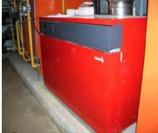
**Figure 7.83. Old generation boiler (140 kW). Figure 7.84. New-generation boiler (300 kW).**
