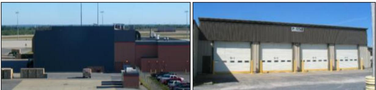
**Figure 7.131.** Left, the completed SolarWall system at Fort Drum's Bldg. 207; right, Bldg. 1750.
