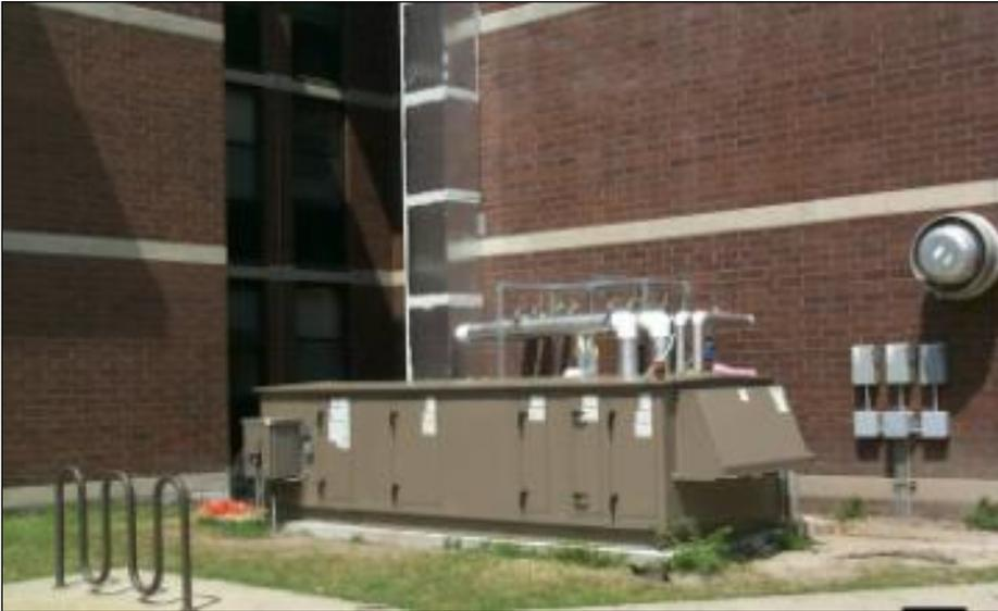
**Figure 7.64. Conditioned outdoor air is ducted from the DOAS AHU up the side of the building to the attic.**
