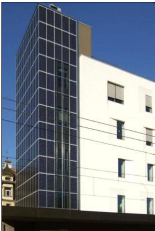
Figure 7.14. View of the PV cells installed on the tower.
