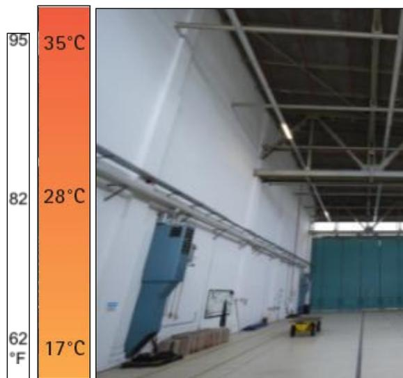
Figure 7.104. A forced-air system was used to heat the hangar.
