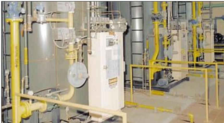
**Figure 7.157. Steam metering at the CRC.**
