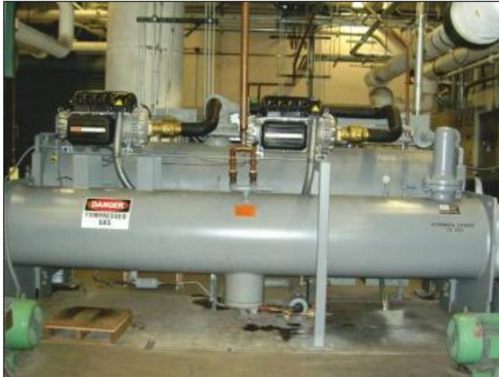
**Figure 7.138. New compressor retrofitted to existing frame in San Diego, CA.**
