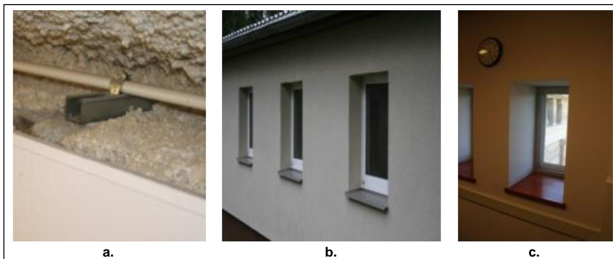
**Figure 6.170. Retrofitted Army barracks with exterior insulation (a), interior insulation of the retrofitted administrative building at the Rock Island Arsenal (b, c).**
