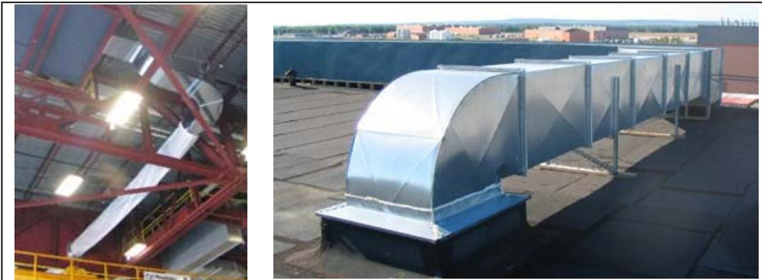
**Figure 7.133. Ventilation air distribution ducting.**
