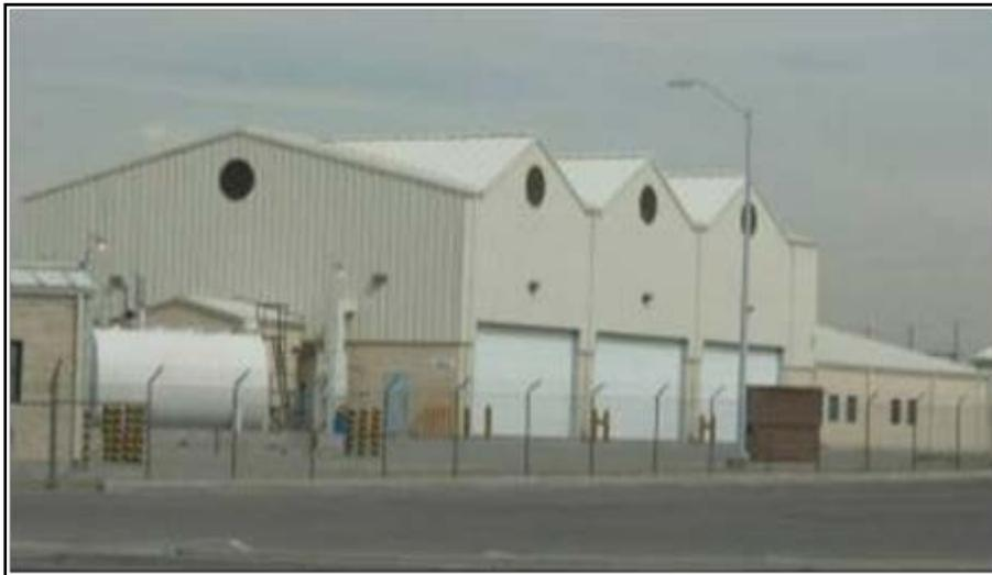
**Figure 6.1. TEMF building at Fort Bliss with a reflective white metal roof.**
