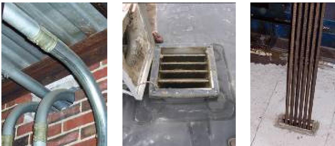
**Figure 6.119.** Unsealed penetrations (left); open louvers to vent shafts (middle); elevator cable holes can be made tighter (right).
