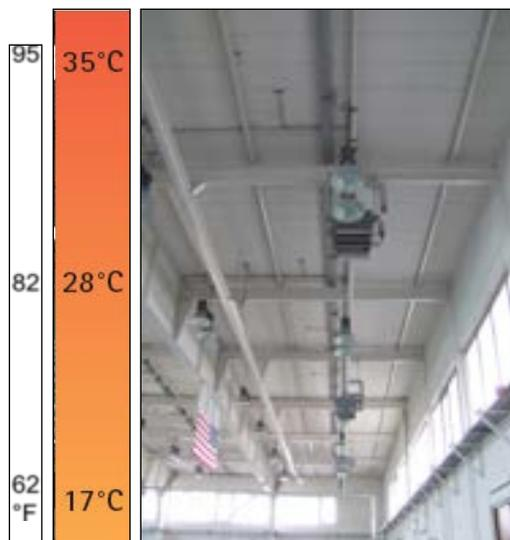
**Figure 7.121.** A forced-air system was used to heat the hangar.
