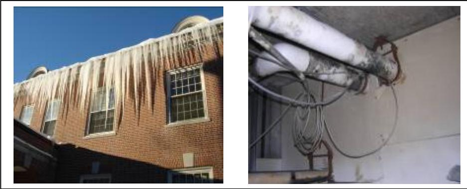
Figure 6.164. Cold climate exfiltration problems (left) and hot humid air infiltration problems (right).
