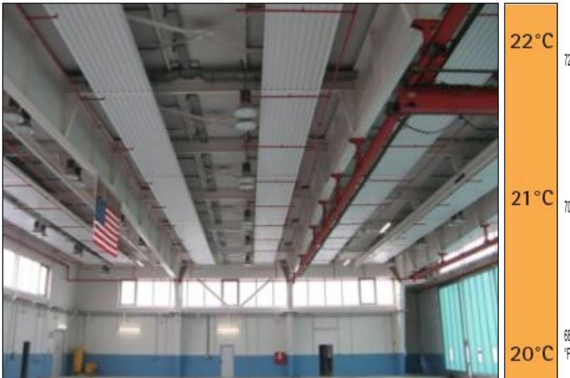
Figure 7.122. The new radiant power heating keeps the temperature more constant between the floor and ceiling.
