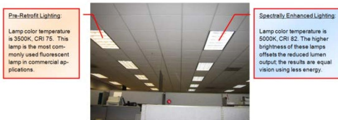
**Figure 6.83. Warm color lighting on the left, spectrally enhanced lighting on the right.**
