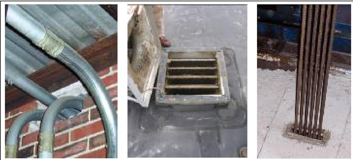
Figure 6.166. Unsealed penetrations (left); open louvers to vent shafts (middle); elevator cable holes can be made tighter (right).
