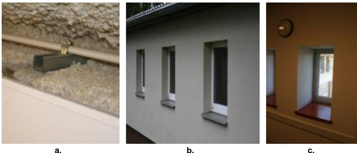
**Figure 6.126. Retrofitted Army barracks with exterior insulation (a), interior insulation of the retrofitted administrative building at the Rock Island Arsenal (b, c).**
