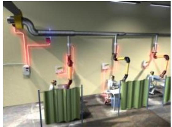
**Figure 6.105.** Demand-based local exhaust system for a typical welding shop.
