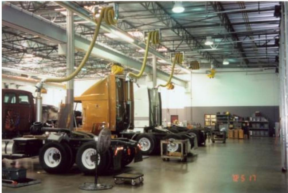
**Figure 6.47. Stationary vehicle exhaust system in the maintenance shop.**
