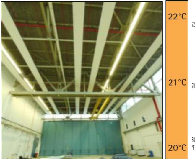
Figure 7.105. The new radiant power heating keeps the temperature more constant between the floor and ceiling.
