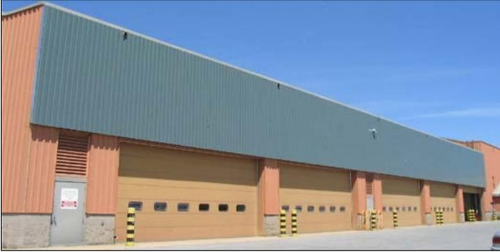
**Figure 7.129. Unglazed SolarWall panels installed above rollup doors of a maintenance shop, Fort Drum, NY.**
