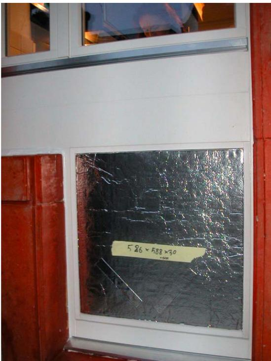
Figure 36: Window element with tight-fitting VIP
