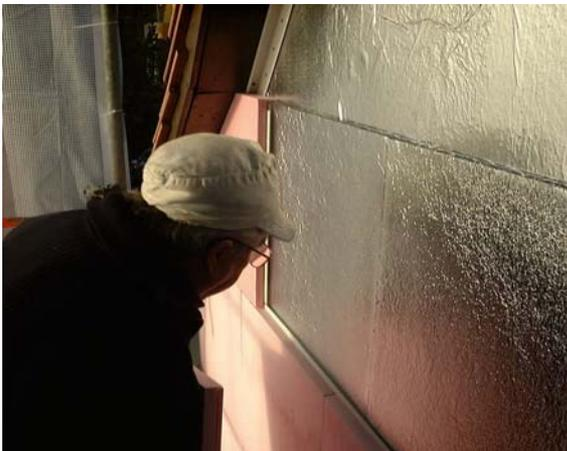
Figure 41: Gable during installation. The shiny VIP are already in the rail system. The pale pink polystyrene boards are being mounted.
