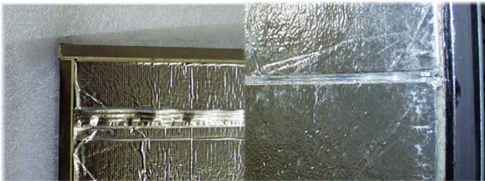
*Figure 57: Gaps and edges of VIP in the elements
