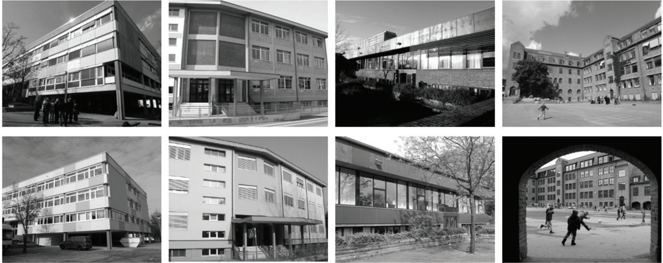
Figure 1 Photos of the four school buildings in the School of the Future project (top row: before retrofitting, bottom row: after retrofitting). From left to right: Solitude Gymnasium in Stuttgart, Tito Maccio Plauto Middle School in Cesena, Hedegårdsskolen in Ballerup, and Brandengen skole in Drammen.
