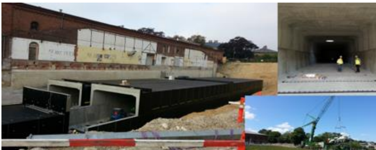
Fig. 3: Chilled water storage under construction
